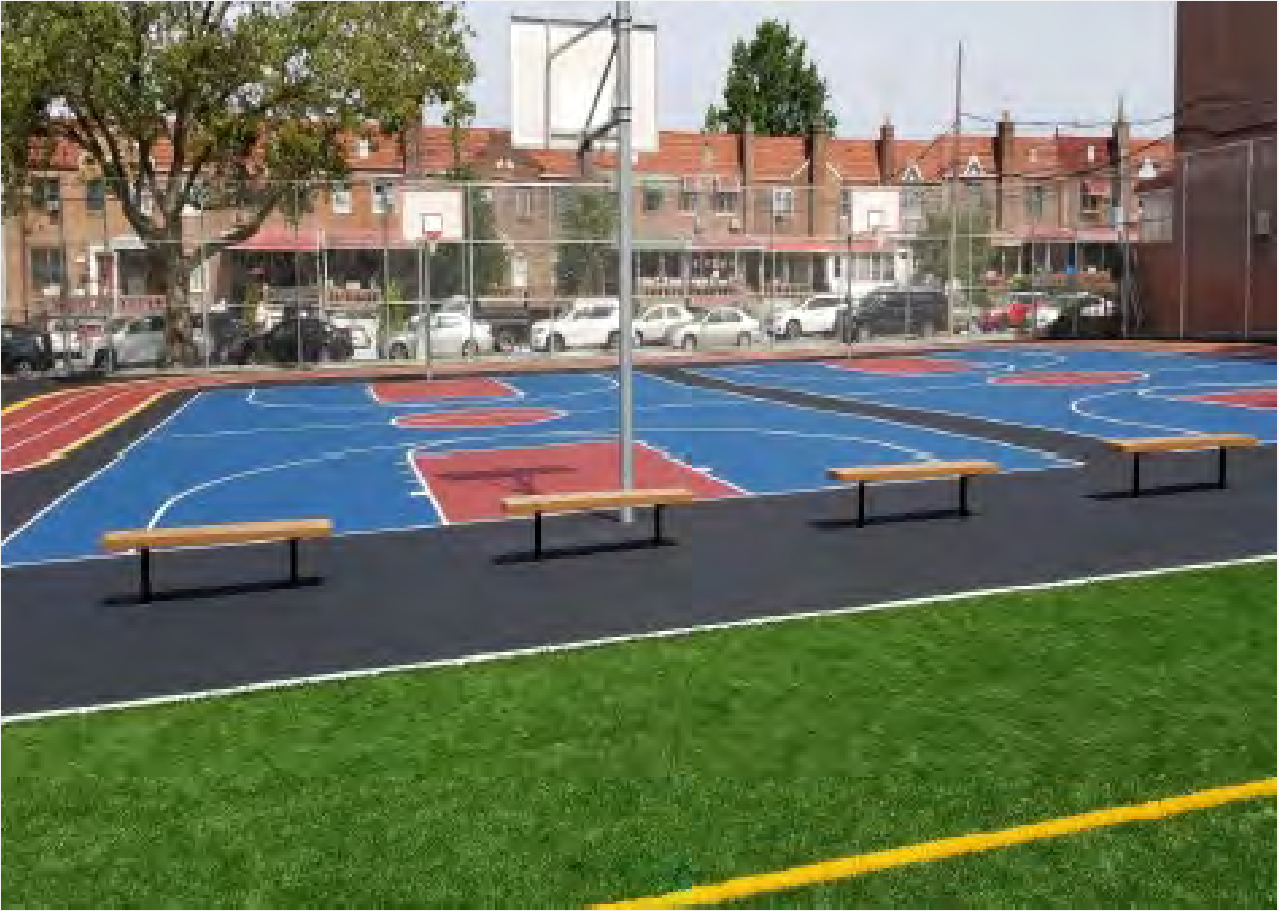
P.S. 151 | TCU Removal & Playground Redevelopment
